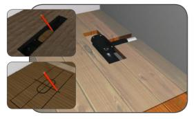
Measure the shower drain base position on the floor and mark this onto the relevant flooring. Using a jigsaw cut a **615mm x 90mm** hole in the floorboard, making sure the drain's centre is in the middle of the cut-out, so that the shower drain base and shower drain connector will be exposed through the new floor.
